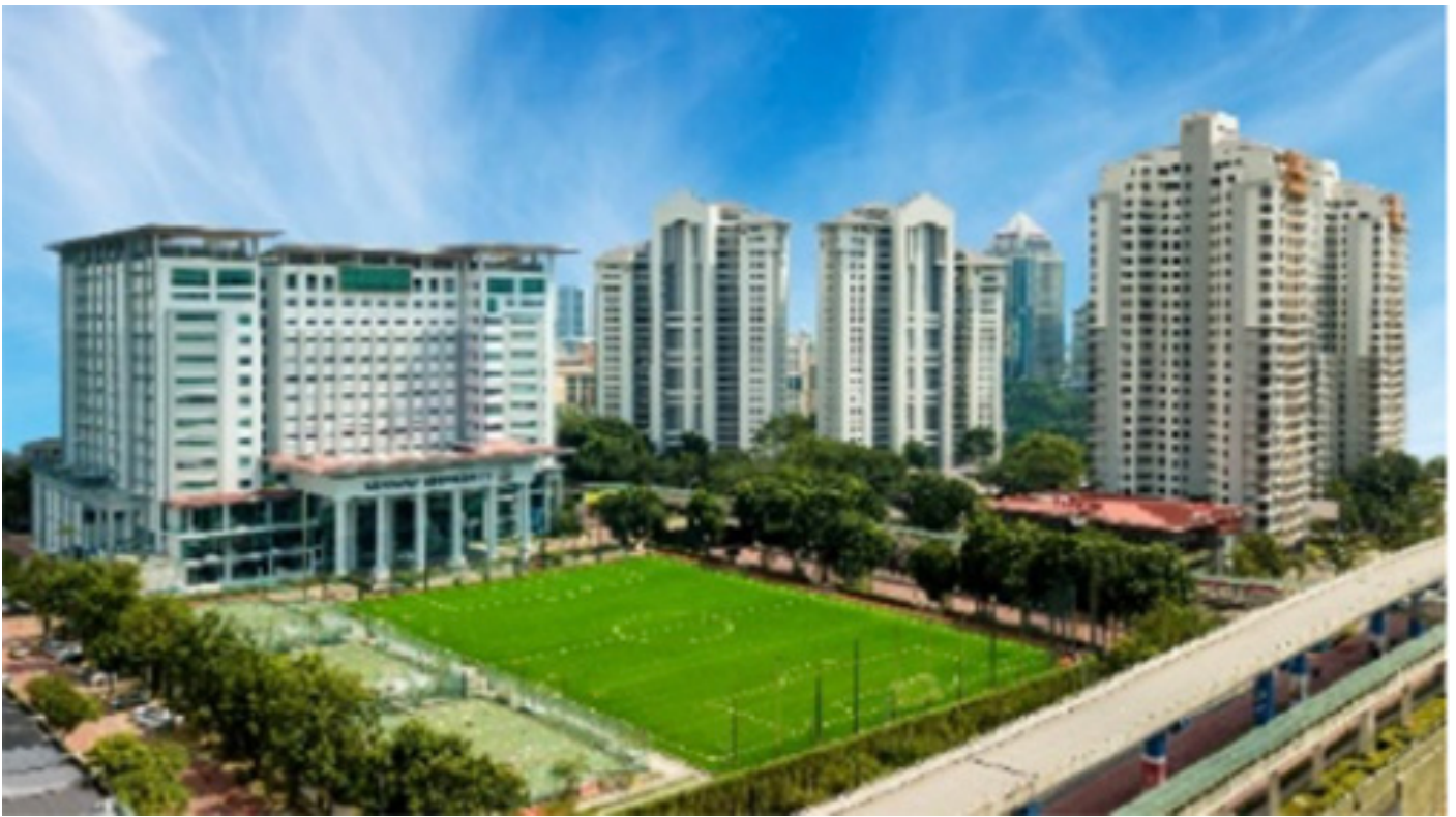
▲ Campus of Sunway University, Malaysia. Source: https://university.sunway.edu.my/about-us .
