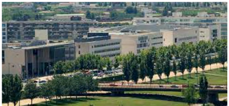
▲ View of Capped Campus of University of Lleida .
